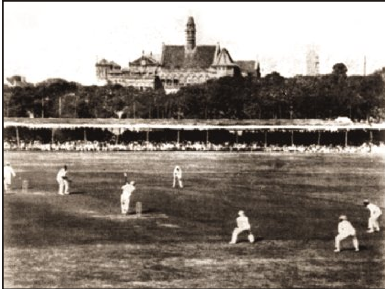
A view of the Bombay Quadrangular 1927.
